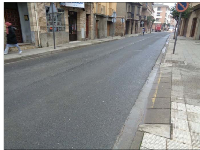
TRAMO MERCED A C/ GOYERA
