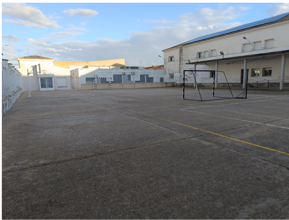
Vista general del patio (22-10-2025)
