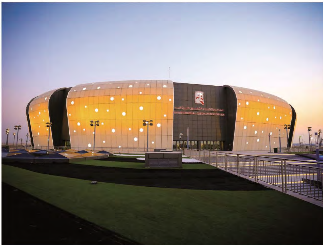
Qatar Handball Association Complex, Doha, Qatar
