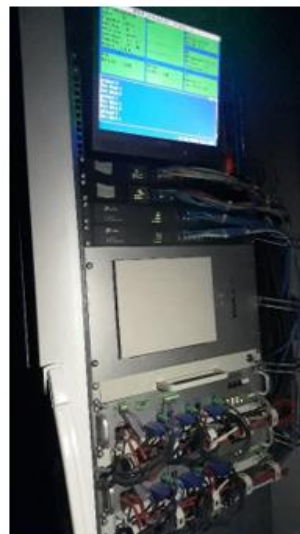
Armario principal de control: ShowController
